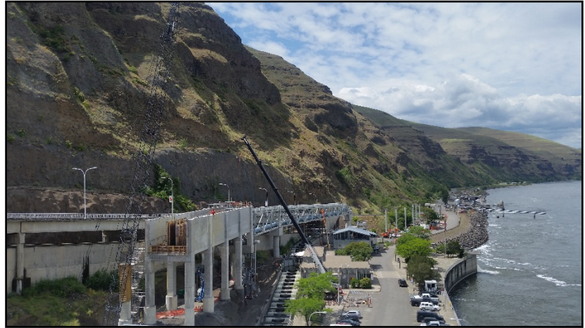
Lower Granite Juvenile Bypass System elevated flume under construction. It will lead fish to the downstream Juvenile Fish Facility. US Army Corps of Engineers photo.
